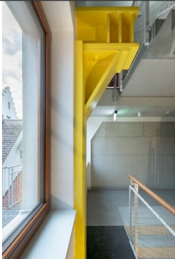
3) Integrated existing steel structure, © Nina Baich 4) Seminar room, © Nina Baich
