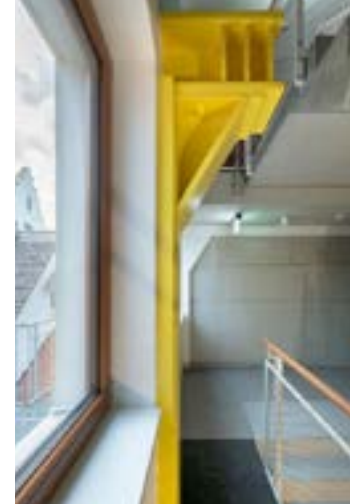
3) Integrated existing steel structure, © Nina Busch 4) Seminar room, © Nina Busch
